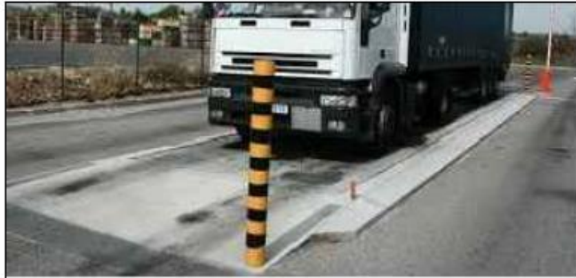
TYPICAL WEIGH BRIDGE 100 TONNE CAPACITY
